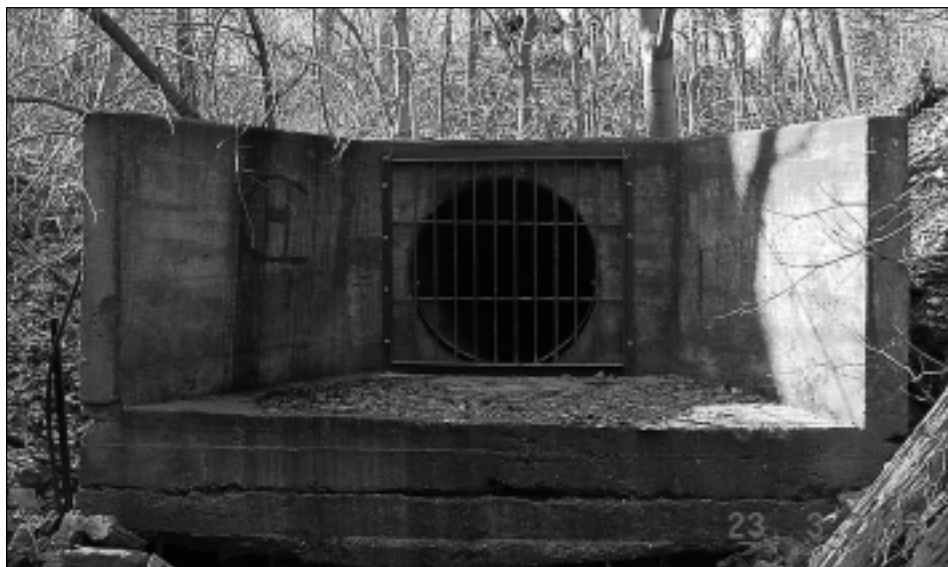
The CSO at Sterling and Forsyth has on average 30 overflows a year, totalling about 52,000 cubic metres.
